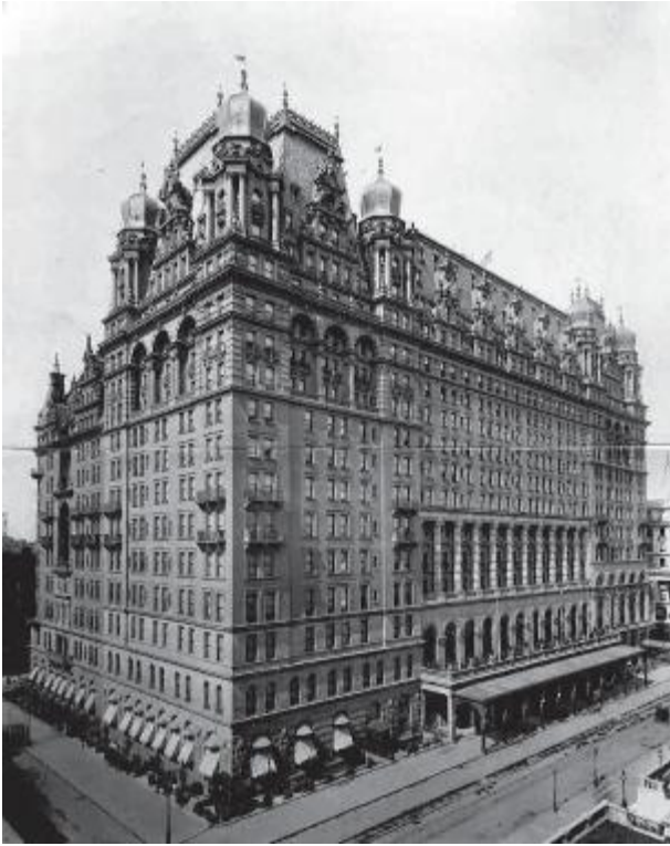
Hotel Waldorf Astoria. (The Hotel Waldorf-Astoria, New York, N.Y., American Architect and Building News, 27 agosto 1898, v. 61, pl. 1183).
