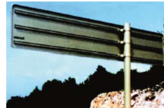
Photo 11. Perimeter reinforcement with a double bracket
