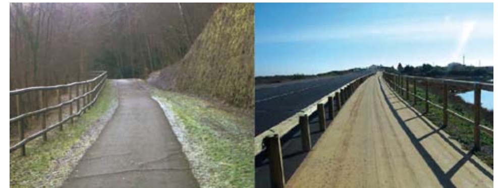
Photo 16. Wooden containment barriers on cyclepaths
