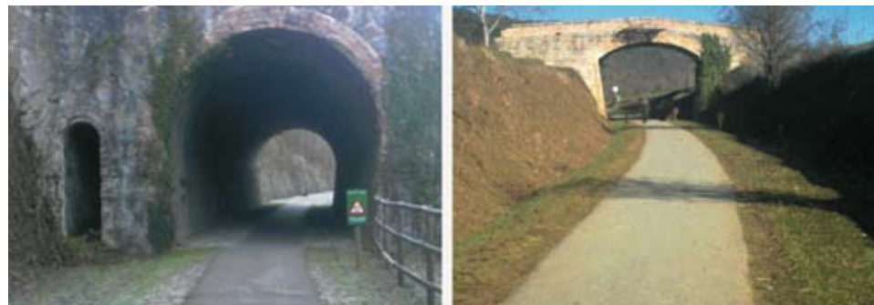
Photo 5. Underpasses on the cyclepaths
