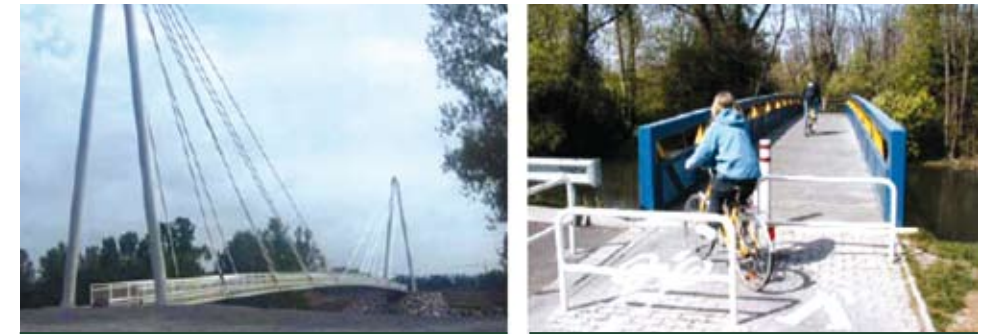
Photo 4. Footbridge for cyclists
